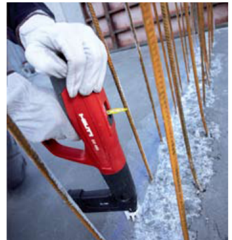
X-FS Form Stop being installed.
