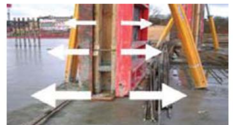
Outward pressure increases towards the bottom.
