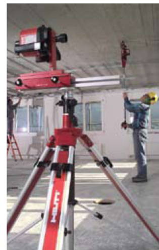
PR 25 laser combined with DX cartridge Tool on Pole Tool.
