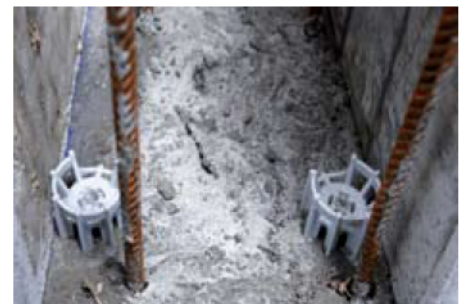
Form Stop locates inner face of form work.
