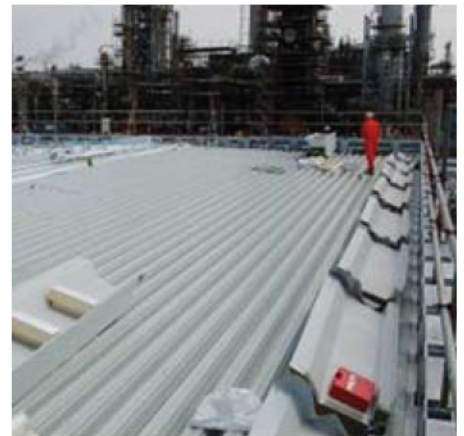
Liner Tray fixed to structural steel.
