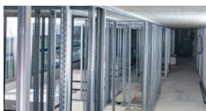
Drywall tracks to concrete and steel
