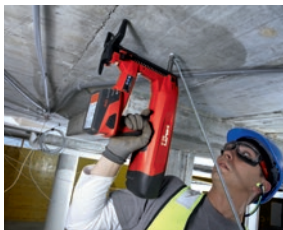
Threaded rod attachments to concrete
